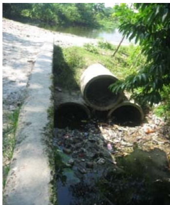
Figure 4: Solid waste accumulation at sewer outfall on the Mayur River, Chhoto Boyra (Shashan Ghat).
